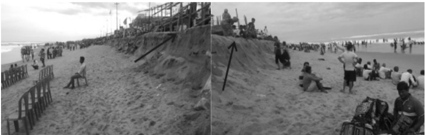
Figure-I Coastal Erosion at Puri, near to the Beach Road at Swargadwara (17.08.2016; 16.20Hrs)
